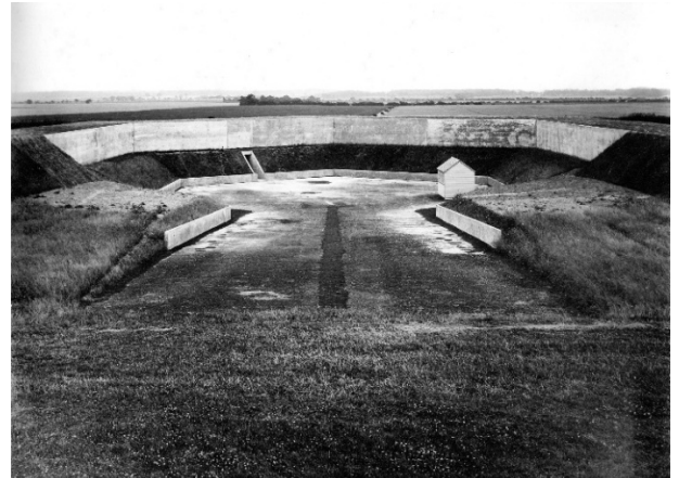
Blast-proof bombing-up pit, Feltwell, 13 July 1939. (credit: M.W. Buckley collection).
